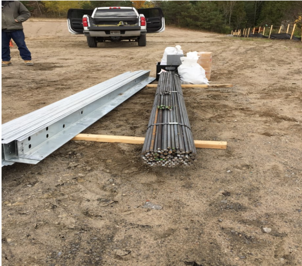
PRE-FABRICATED DIMENSIONALLY STABLE EXTERIOR FORM CHANNELS WITH PRE-DRILLED PERIMETER BEAM BAR AND SLAB GRID BAR SLOTS
